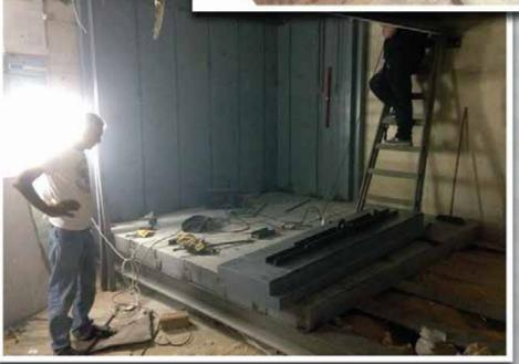
Construction of a vault room in an existing building. The walls are build with ISM's anti burglary modular panels.
