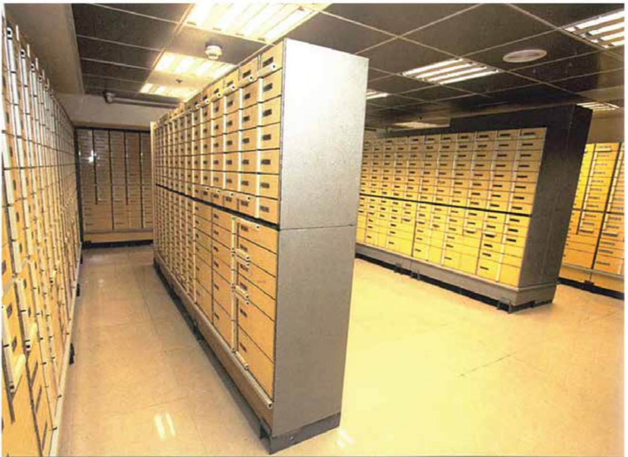
Vault Room of an Israeli Bank
